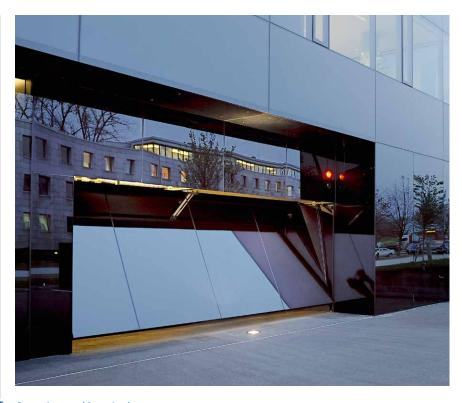
Gas springs enable optimal gate movement.
